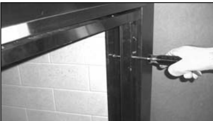
Figure 10.3 Loosen Refractory Retaining Strip
