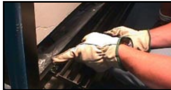
Figure 23 - Replacing the Control Access Panel
