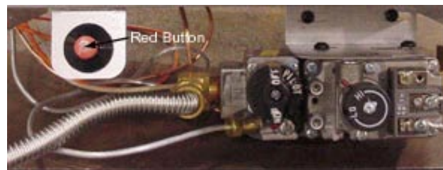
Figure 24 - Standing Pilot Ignition
