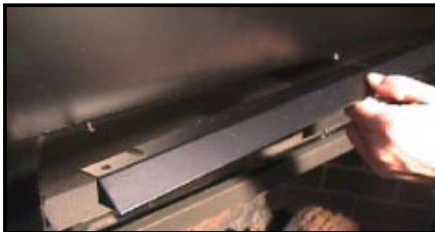
Figure 18 - Hood Placement
