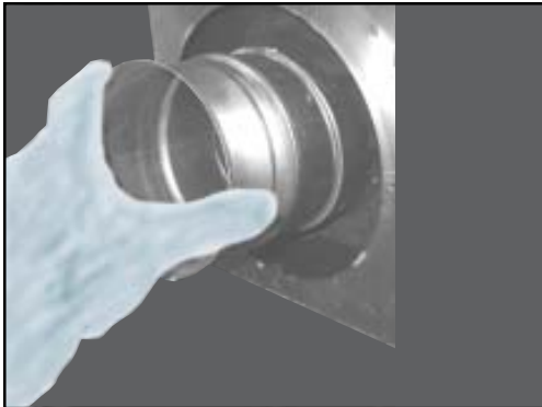
Figure 8.7 Insert inner collar adapter to rear flue vent.
