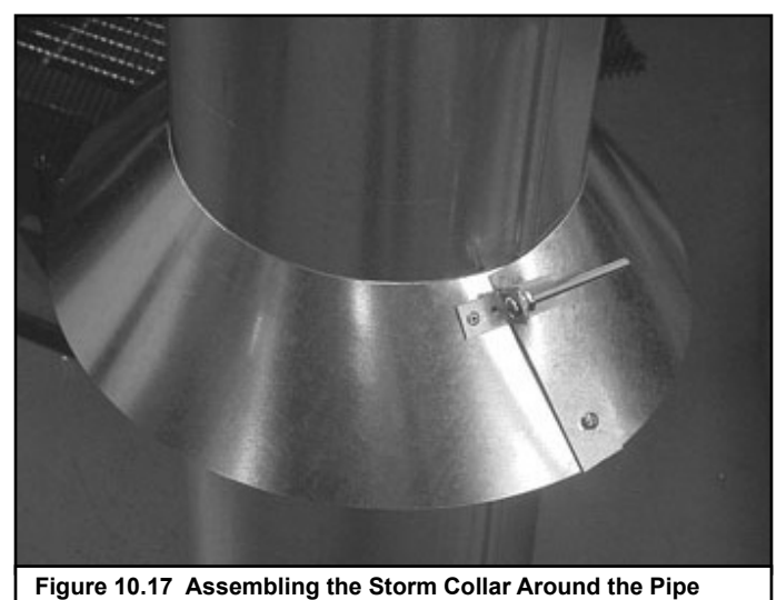
Figure 10.16 Assembling the Storm Collar
