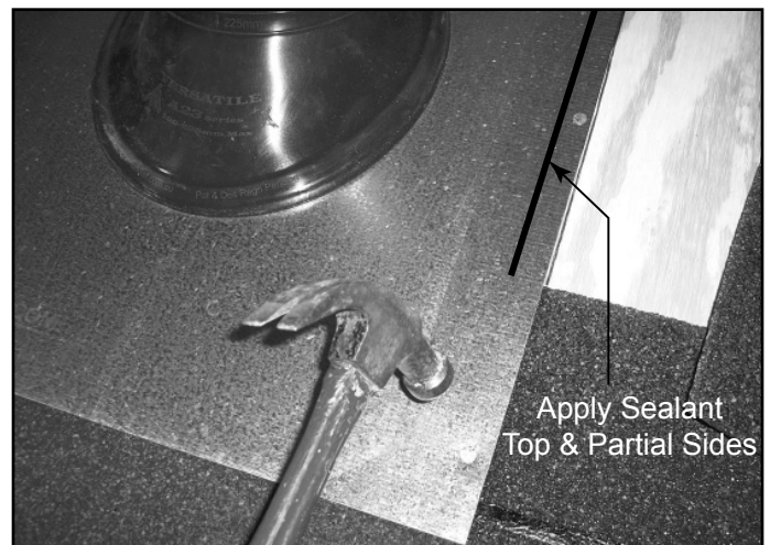
Figure 10.21 Slide Flashing Down, Secure & Apply Sealant
