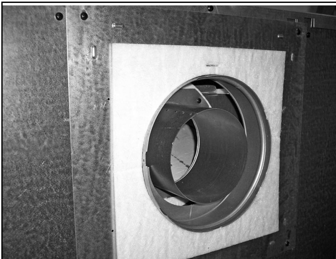
Figure 9.13 Place Insulation over the Cover Plate
