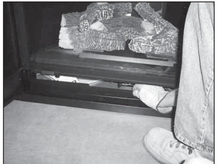
Figure 15.11 Installing Floor Cover
