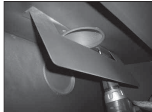
Figure 7.7b Remove Flue Visor
