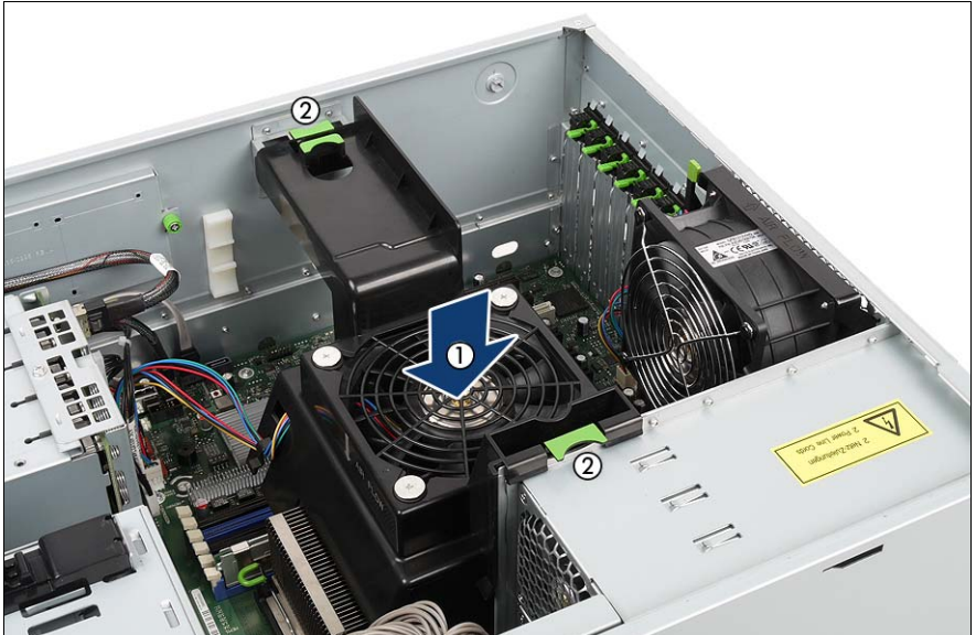
Figure 37: Installing system fan 2 (and 4)
