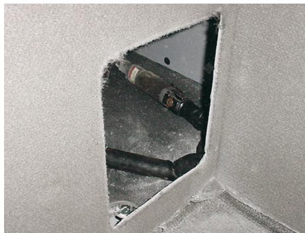
Figure 9 - Return air vent hole cut
