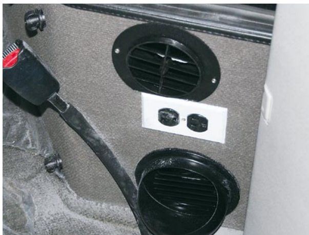
Figure 17 - 4" ducts installed low on the floor on the driver's side
