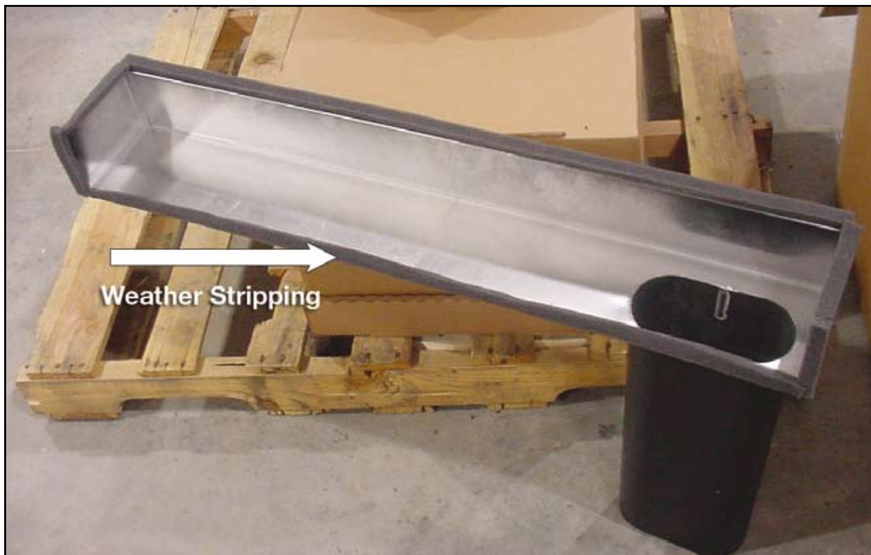
Figure 9. Installing the weatherstripping on the custom plenum.
