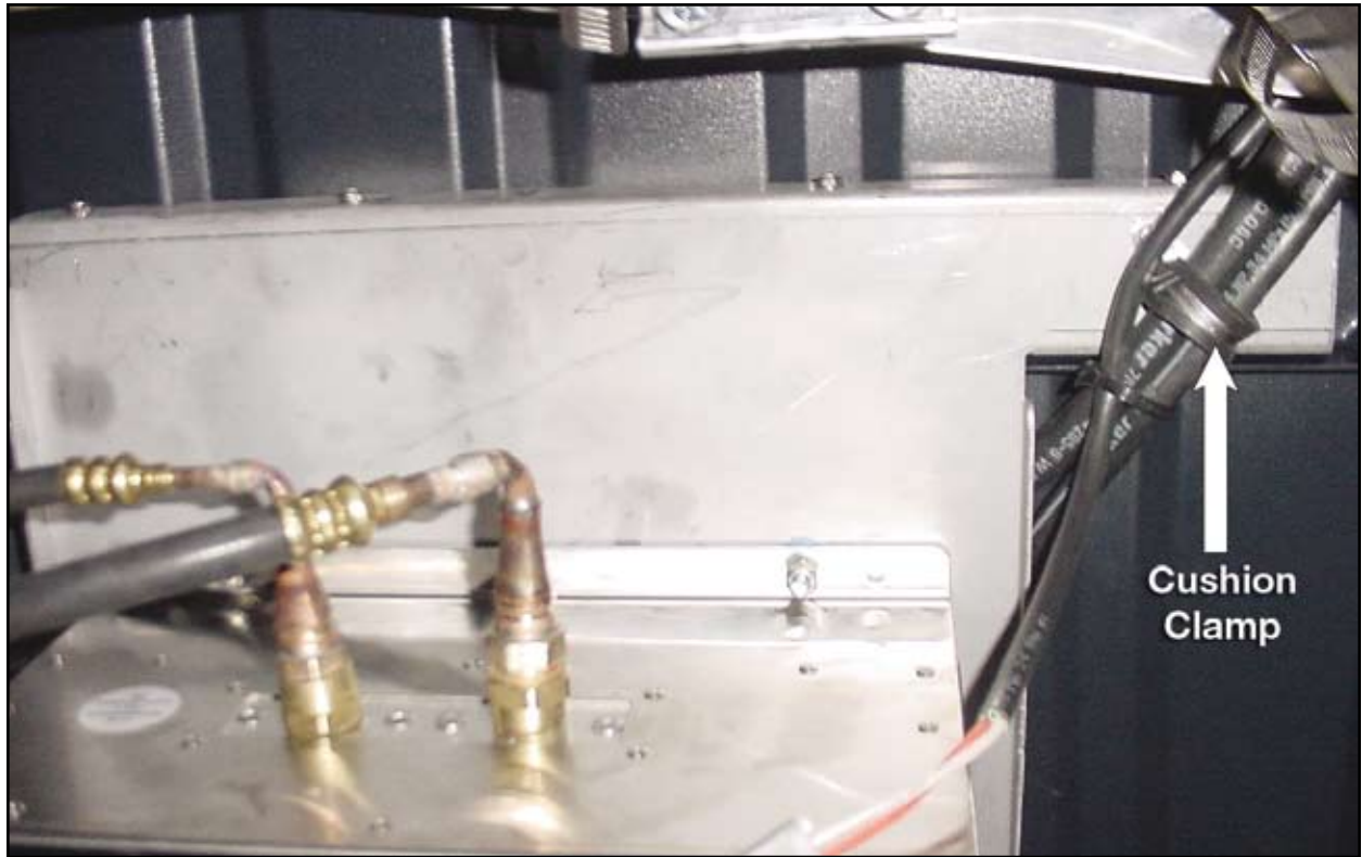
Figure 17. Routing of refrigerant lines.
