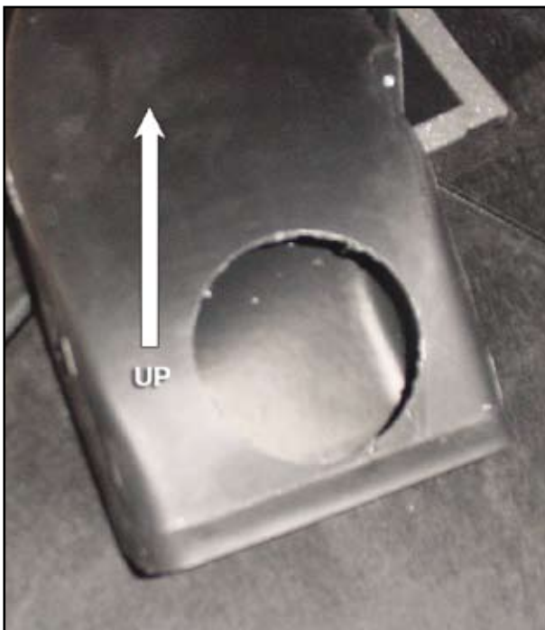
Figure 8a. Four inch hole cut in Volvo duct.
