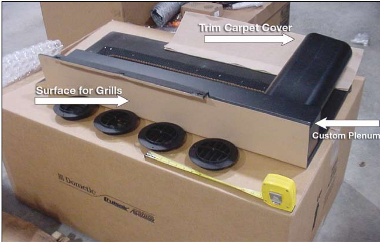
Figure 10. Preparing to install grills in footwell cover.
