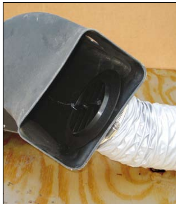
Figure 8b. Installation of grill and ducting.
