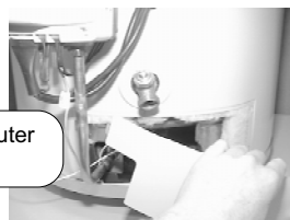
Slide inner door open from left to right.
