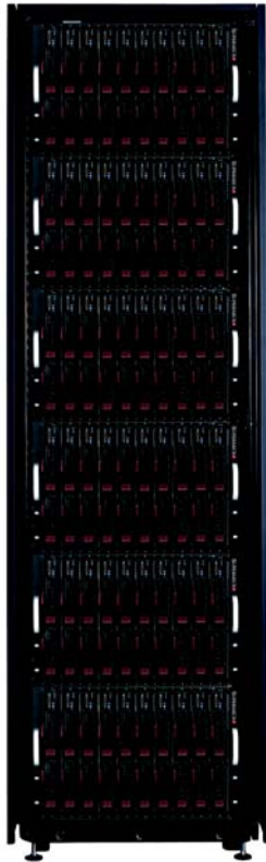
Figure 1-1. Full Rack of Blade Enclosures and Blade Servers
