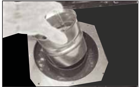
Figure 8.2 Remove the inner collar adapter.
